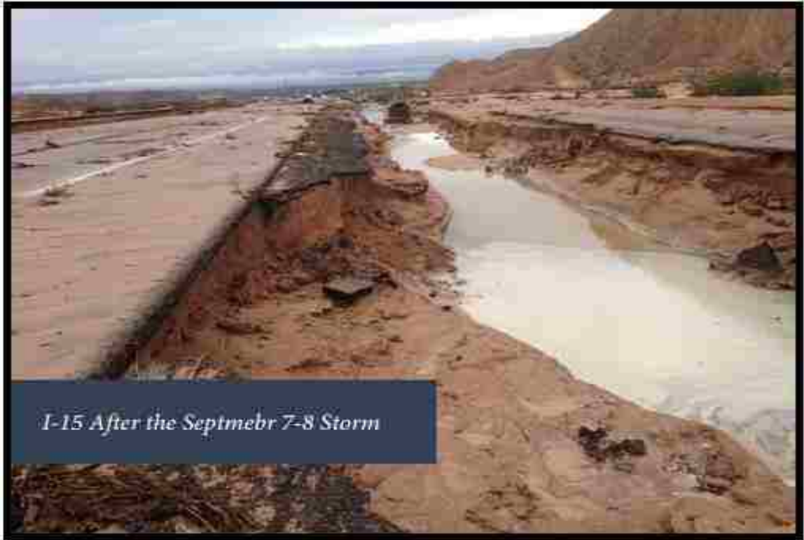
Figure 2.5-3: Photo of a damaged section of I-15 due to the flood events of Sep 07, 2014. (Source: CCRFCD)
